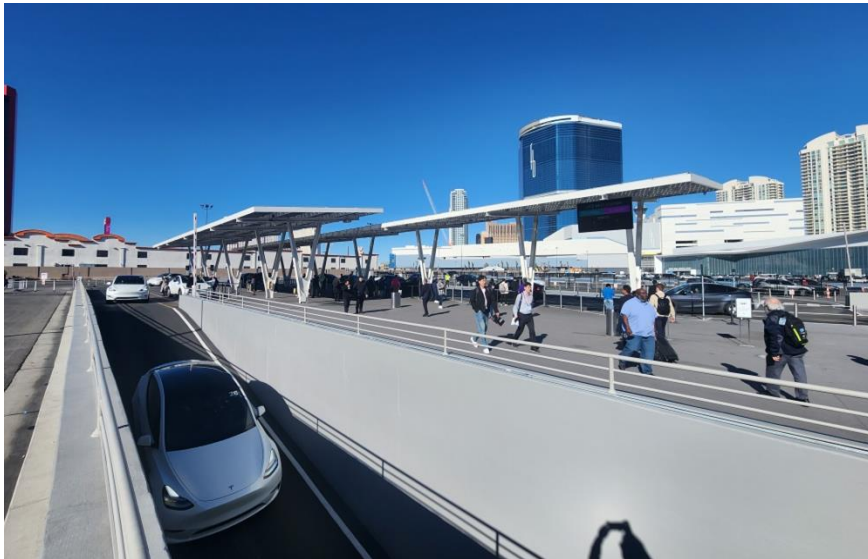
Boring Company LVCC West Station
