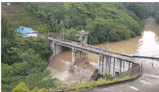
Hydropower Plant in Indonesia
